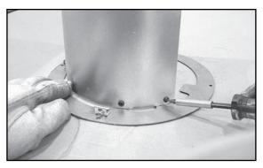
Figure 5.33 Attach the heat shield to the trim ring with the four screws provided. Screws go through the heat shield and into the brackets on the trim ring.
